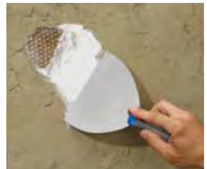
Quickly repair holes in drywall or plaster: 3M™ Patch Plus Primer Spackling Compound
